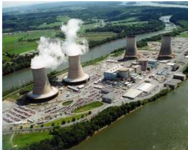
Three Mile Island (TMI) Nuclear Power Plant
